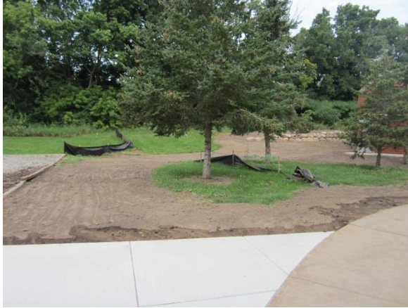
The exterior of the west side is ready for landscaping.
