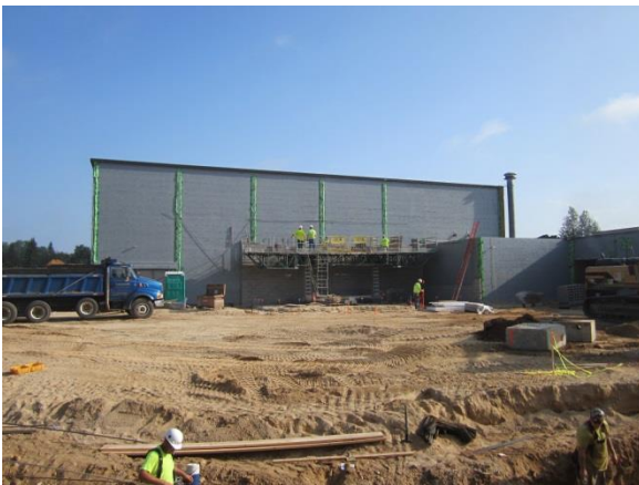
The "Living Wall" is nearing completion. This will provide slope stability with vegetation growing on it at the Pheasant Branch Conservancy.
