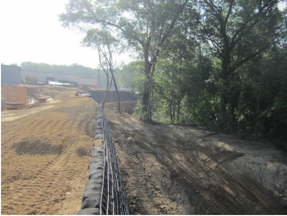
The "Living Wall" is nearing completion. This will provide slope stability with vegetation growing on it at the Pheasant Branch Conservancy.
