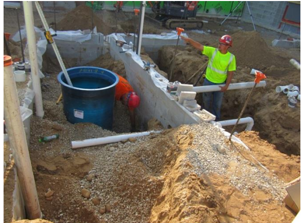
Underground plumbing is underway in the 5 th grade wing.
