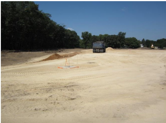
Site grading continues where the football field was.
