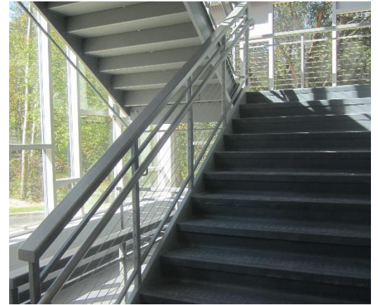
Stairs are complete – Areas A & B
