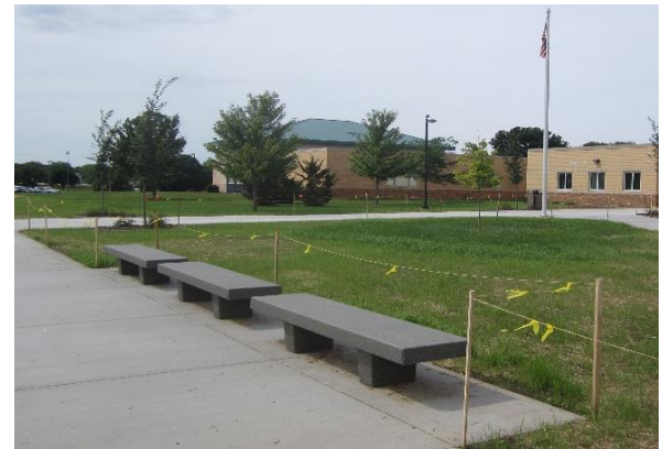
Concrete benches have been placed along entire site - Site
