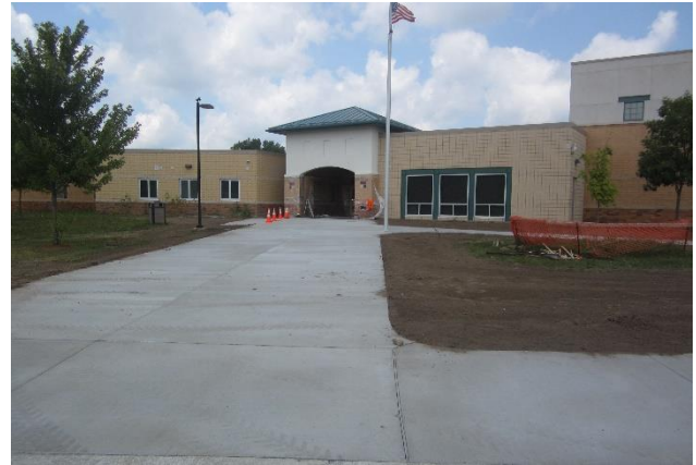
Concrete sidewalks have been poured at the main entrance – Site/Area C
