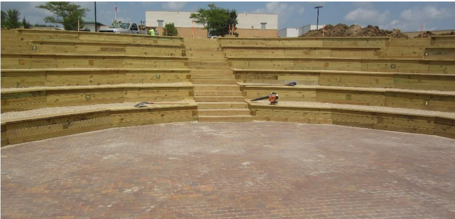
Pavers are in place at the base of the amphitheater - Site
