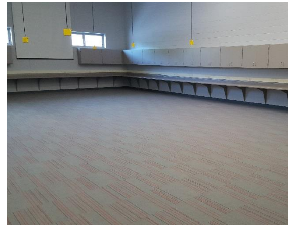
Final product in one of the new GTT rooms!
