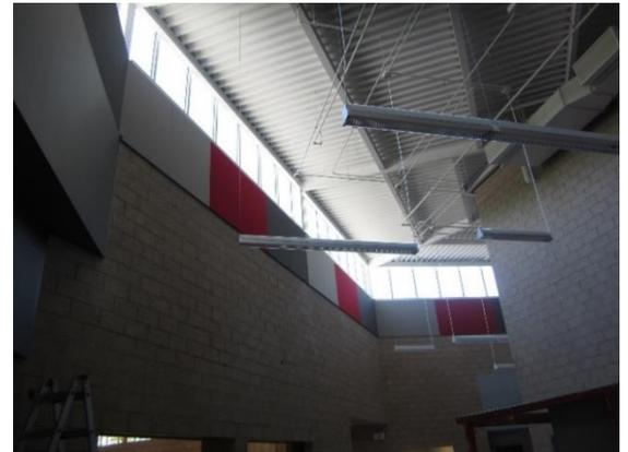
Sound absorbing wall panels, lights, and various other finishes are being installed in the main entrance and corridors – Area C
