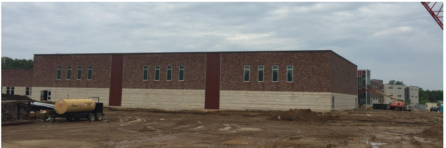
The new athletic field is ready for topsoil to be spread.
