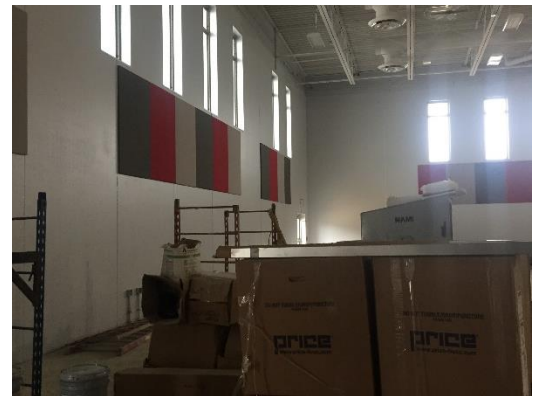
Acoustical wall panels installed in the Fieldhouse
