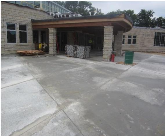
Concrete sidewalks have been poured near the front entrance. Storefront and curtain wall entrance framing and glass installation is ongoing - Site
