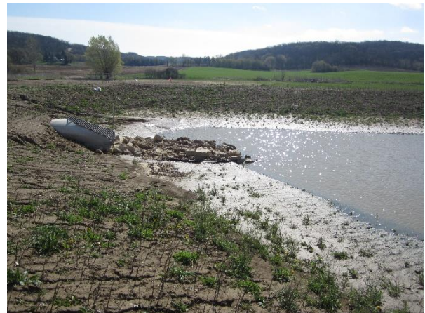
Stone rip-raps are in place in the wet retention area
