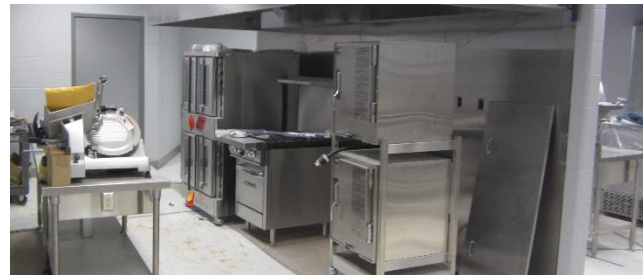
Food service equipment is being installed in the kitchen and servery
