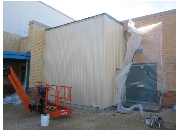
Exterior painting is almost complete.
