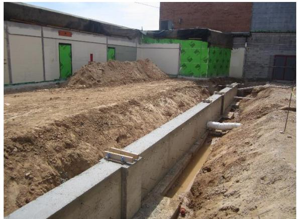
Footings and frost walls for the 5<sup>th</sup> grade wing have been poured – Area D
