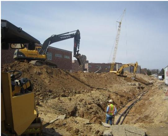
Geothermal trenching and system tie-in is underway
