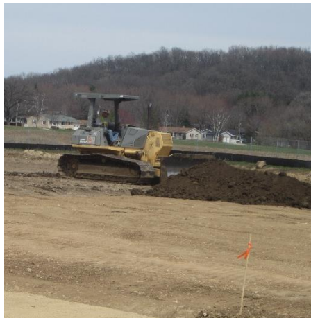
Excavation continues in preparation for the installation of sidewalks and curbs
