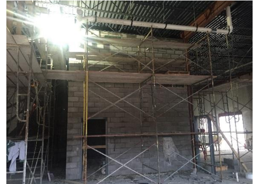
Interior masonry is nearly complete in the new GTT area.
