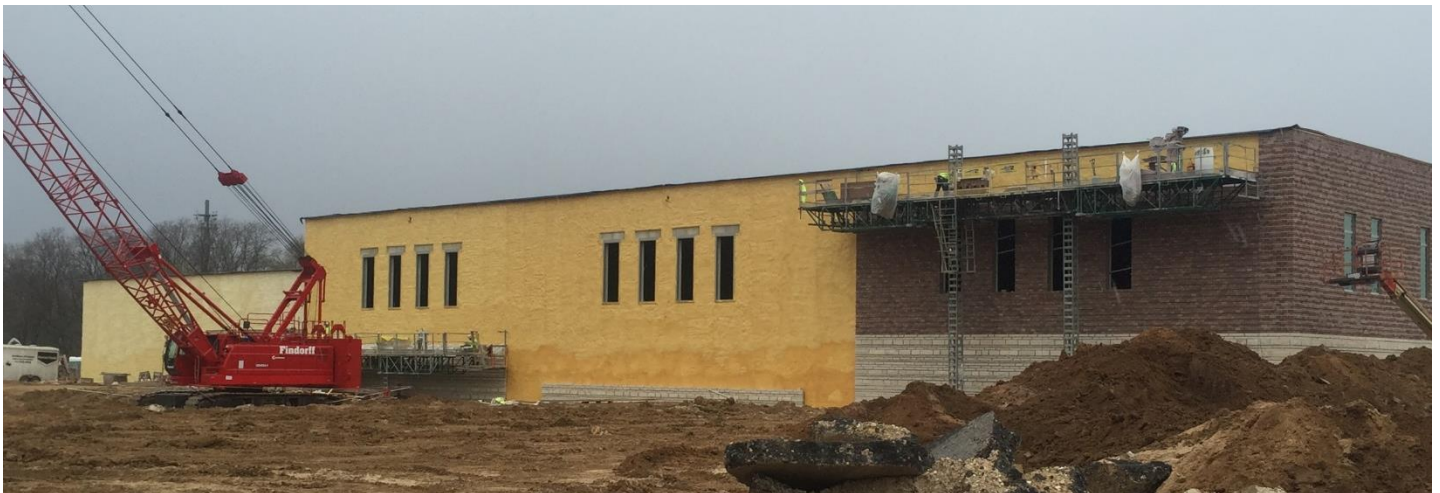
Exterior masonry is progressing around the gym.
