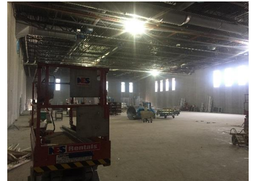
Duct work and electrical rough-ins are underway in the new gym.
