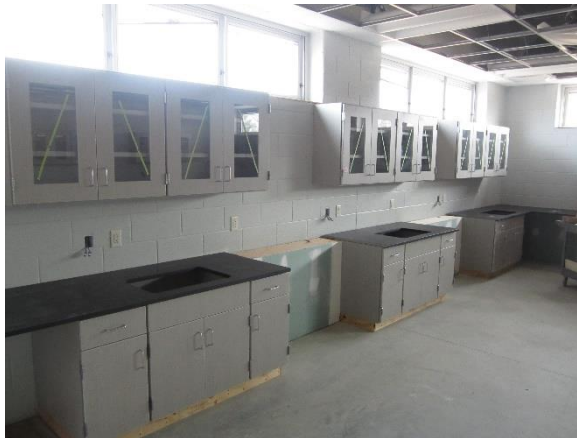
Casework in the 5 th grade classrooms is installed
