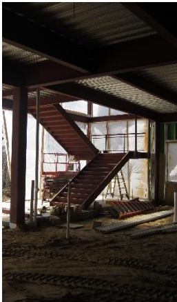
Structure for 6 th , 7 th and 8 th grade stair A-ST1 is in place
