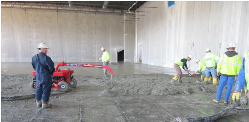
Concrete slab being poured in the new gym.
