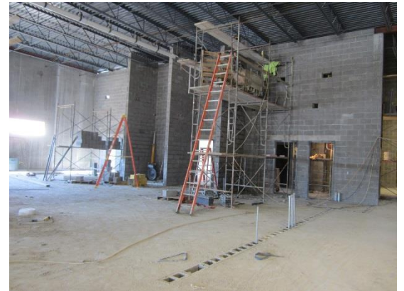
New CMU walls being put up in the GTT area.
