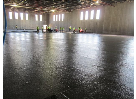
The concrete slab prior to troweling.
