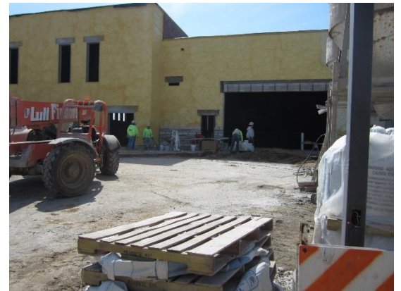
The north side of the building is ready for masonry.
