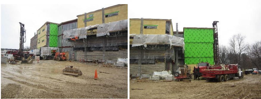
Area A exterior masonry and geothermal well drilling is ongoing.
