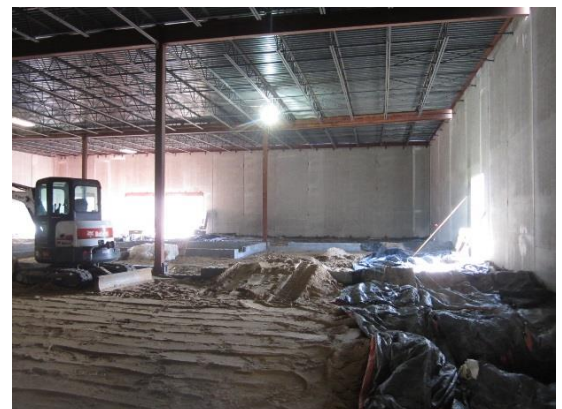
The GTT area is being prepared for slab on grade.
