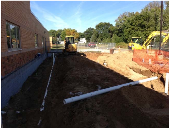
Install Underground Plumbing – Area D (Art & Music)
