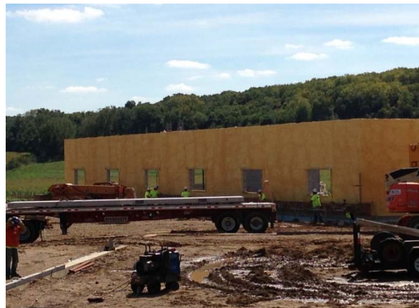
Install Brick Façade – Area G (5 th Grade Wing)
