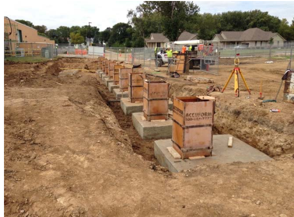
Bus Canopy Foundations
