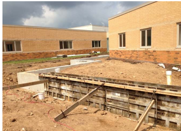
Form and place foundations – Area C (Administration)
