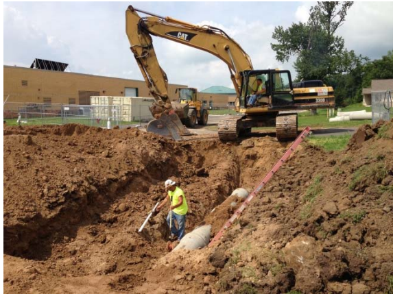
Excavation and installation of site storm drain.
