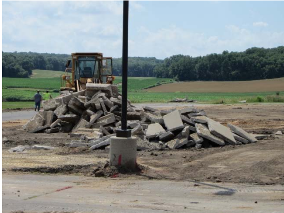
Site clearing in progress.
