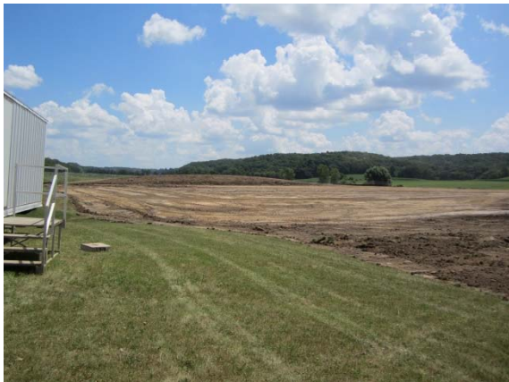
Cutting and filling of site.
