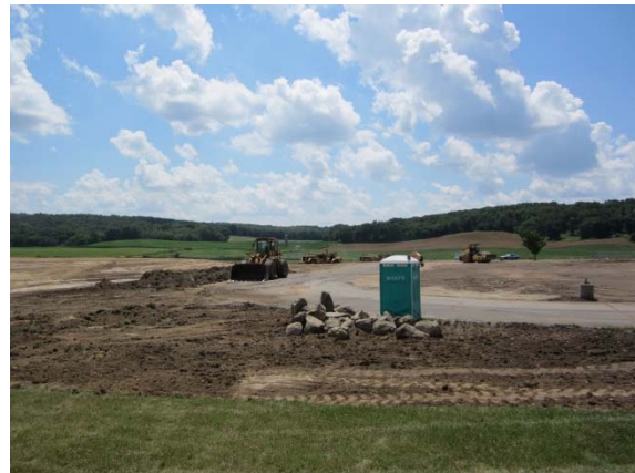
Cutting and filling of site (cont).
