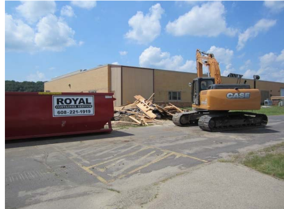
Shed removal in progress.
