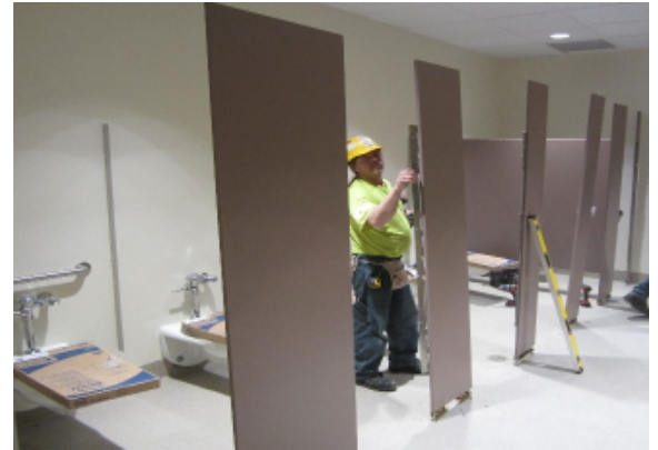
Install Restroom Toilet Partitions – Area F
