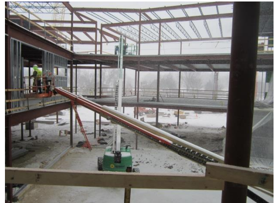
Workers are framing the courtyard of the three story wing.
