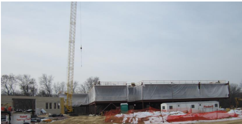
The steel structure of the 6 th , 7 th & 8 th grade wing continues to rise. Plastic sheeting has been installed to allow heating for winter concrete and masonry work.
