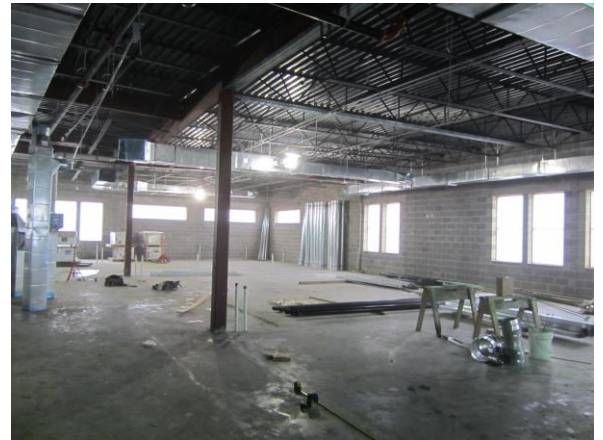
In the 5 th grade wing ductwork and piping rough-ins are underway.
