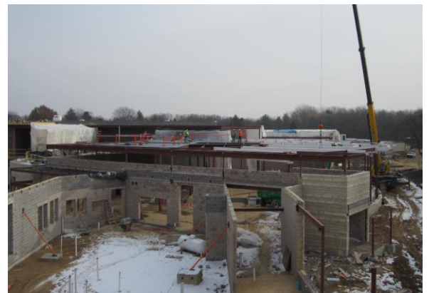
Aerial view looking east over the main office and the cafeteria in the background.
