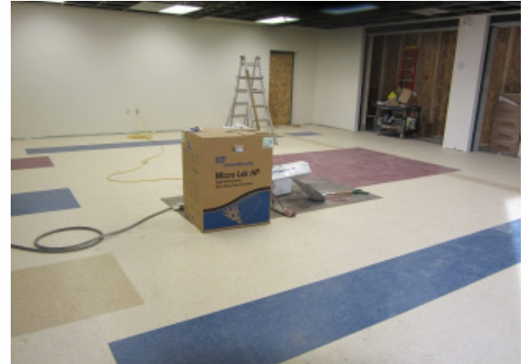
Install Flooring in Commons – Area C
