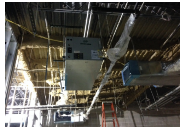
Structural Steel Fireproofing – Area F
