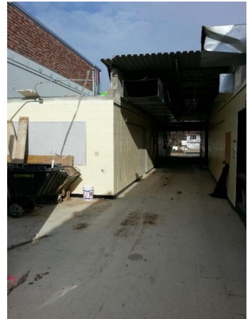
Tech Ed. room and Hallway – Old Building
