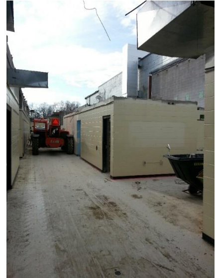
Locker Room Demolition – Old Building
