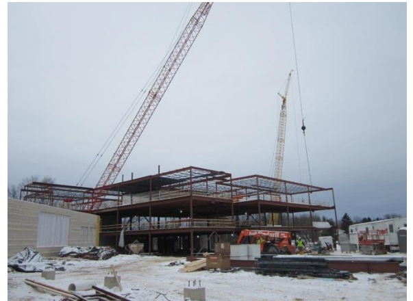
The steel structure of the 6 th , 7 th , & 8 th grade wing is moving west.
