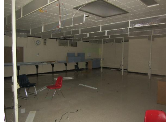
Old building has been vacated – Existing Building
