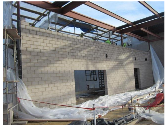
Interior masonry is continuing in the cafeteria.
