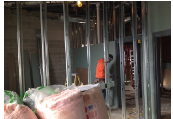
Hang Drywall in Administration Offices – Area C
