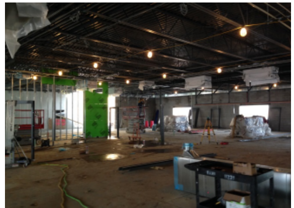
Erect Nano-Wall Supports in 5 th Grade Wing – Area G
