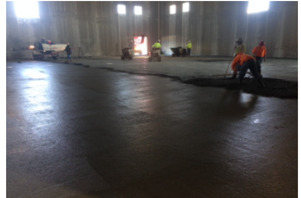
Slab on Grade Placement in Gymnasium – Area F
