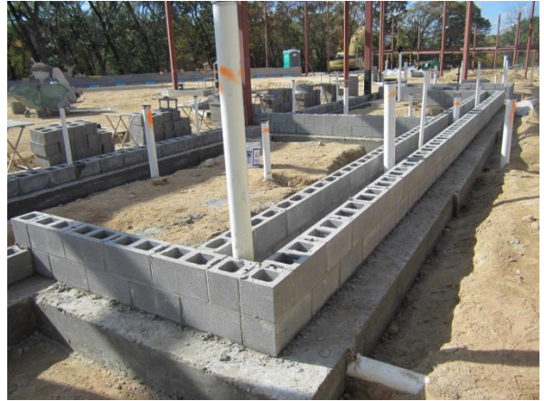
In the cafeteria underground plumbing is being installed for the restrooms.
