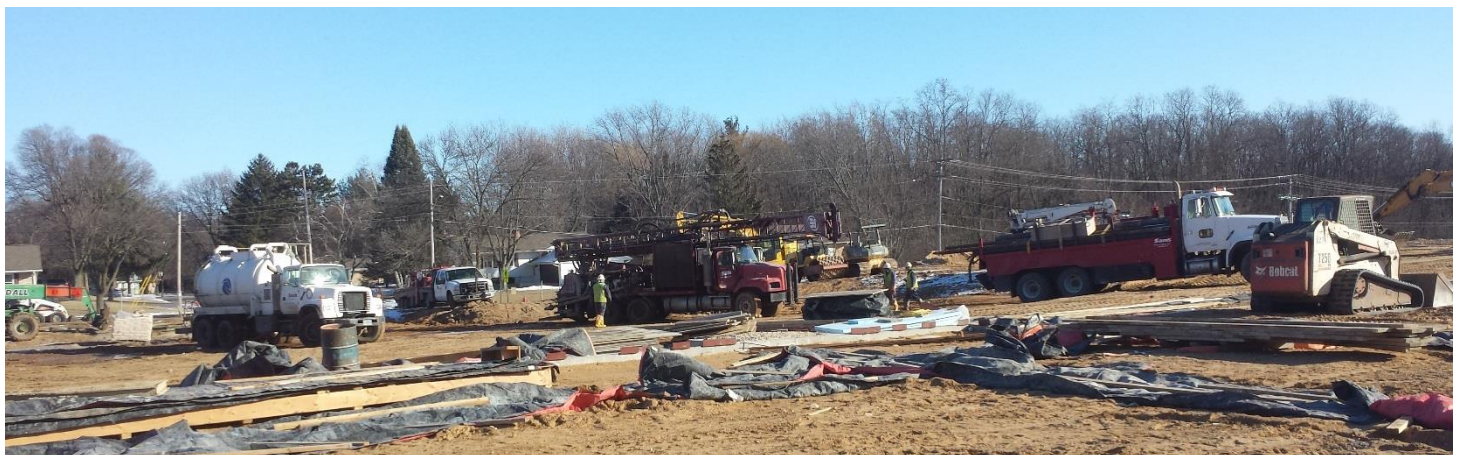
Geothermal well drilling rigs are onsite. A vacuum truck is shown on the left side of the photo for removing drilling fluid, the drilling rig is shown in the center with the mast down.
