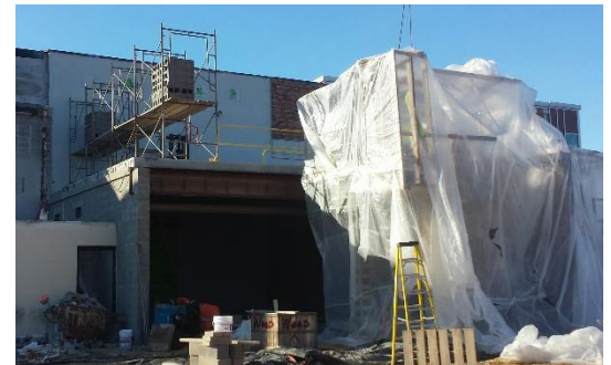
New structure is underway north of the locker rooms.
