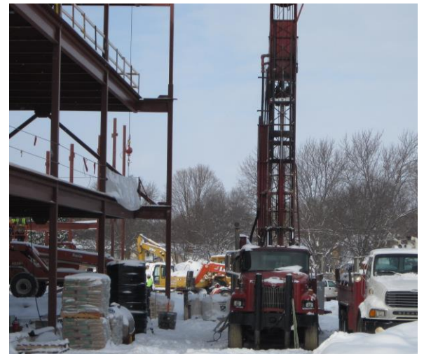
The first drill rig is onsite and boring geothermal wells.
