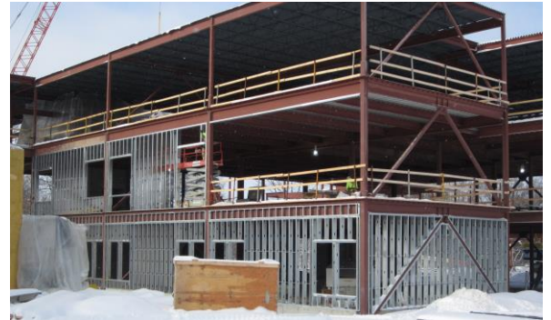
Wall framing on the three story wing is underway.
