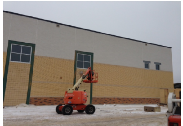
Install Gymnasium Windows – Area F
