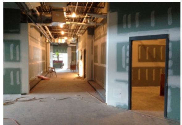
Drywall Finishing – Area G
