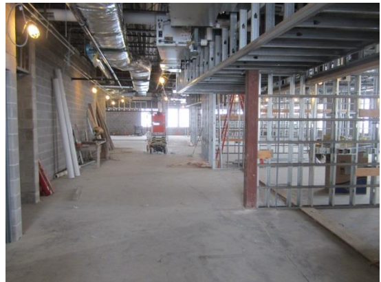
MEP rough-ins are complete in the 5 th grade wing.
