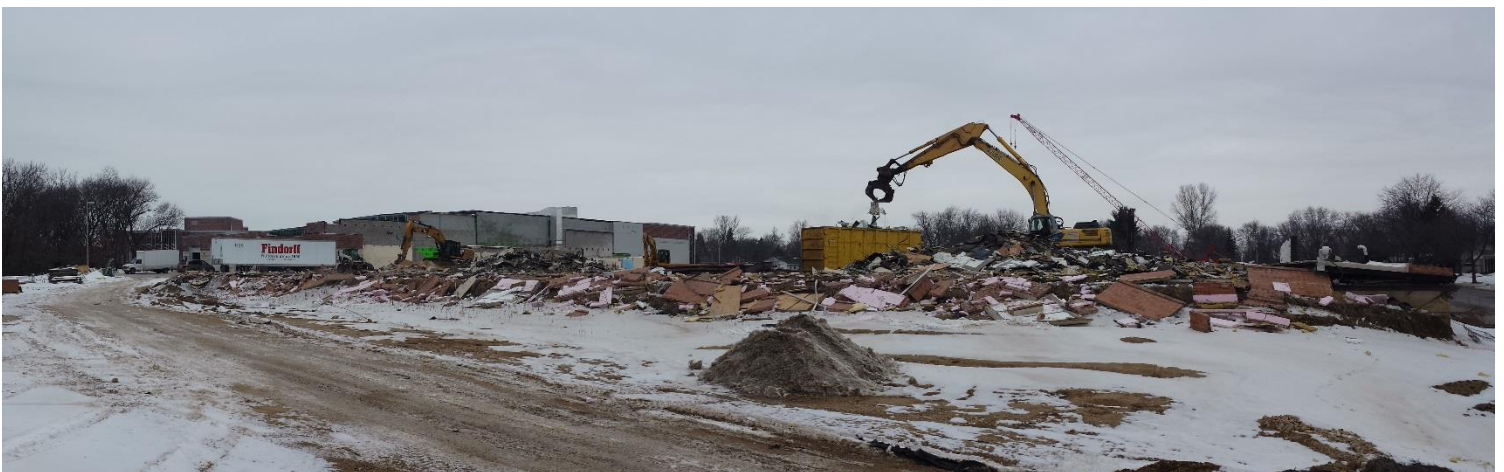
The structure of the old Kromrey is completely down.
