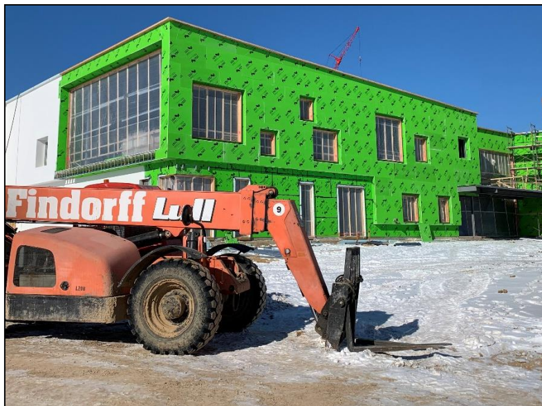
Below: Southeast corner of the building fully enclosed.
