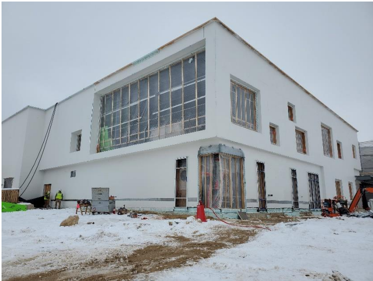
Below: Southeast corner of the building with the white Air Vapor Barrier applied to the building.
