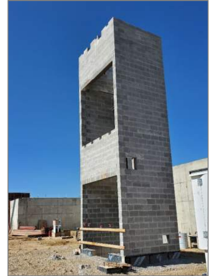
Right: Completed Elevator Shaft Below: North wall of building
