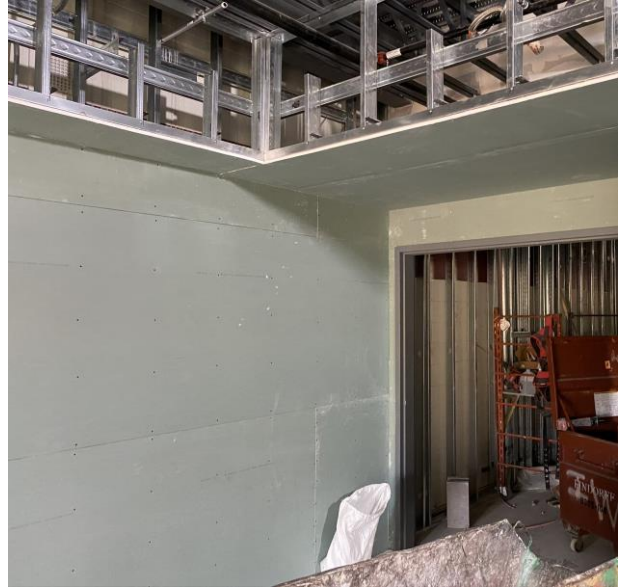
Drywall hung in the concourse vestibule on the first floor.
