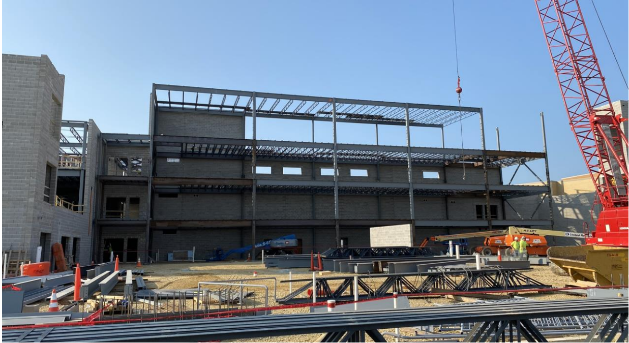
Structural steel continues to be erected in the north addition.
