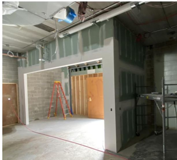
Drywall in the pool vestibule has been mudded and taped.
