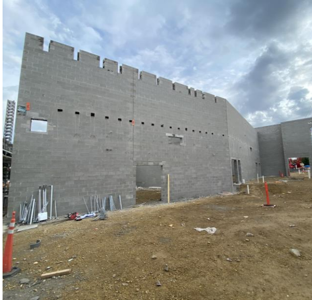
Interior CMU walls constructed in west side of the north addition.
