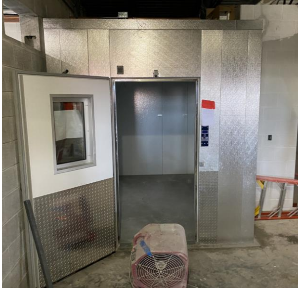
Concrete floor poured in newly assembled freezer.
