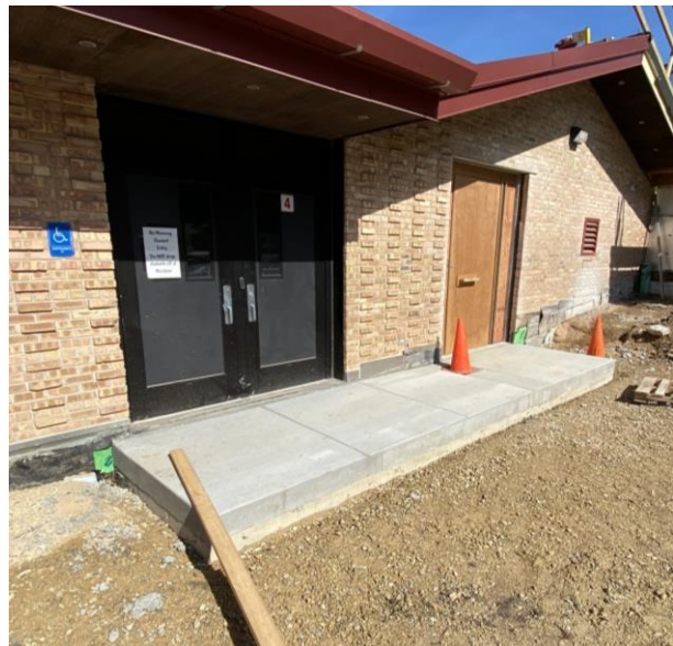
Concrete stoop poured for new receiving room entrance.
