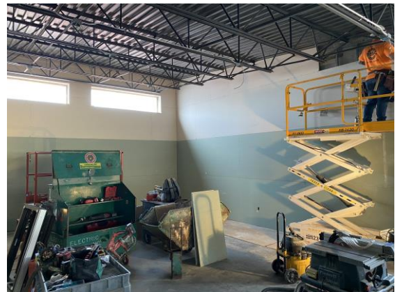
Drywall hung in the cafeteria.
