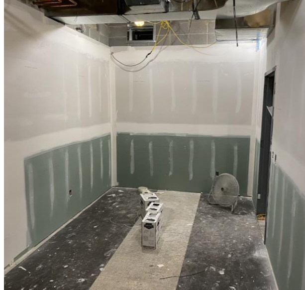
Drywall mudding and taping beginning in the conference room.
