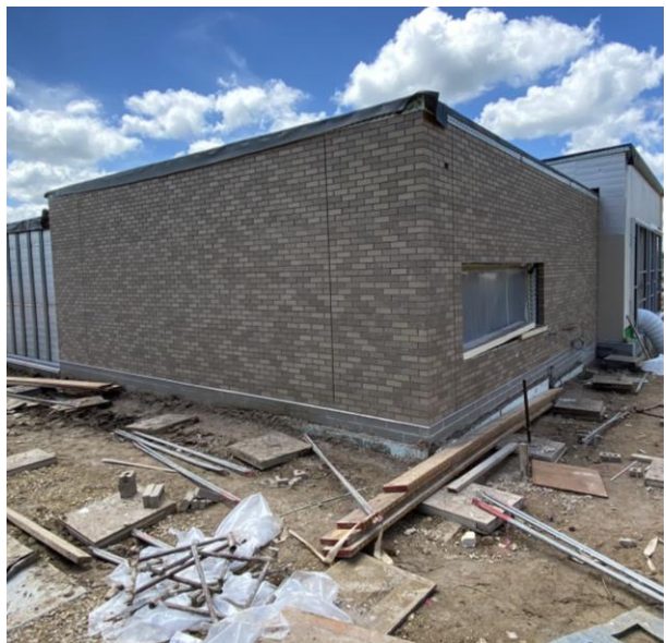
Brick laid along exterior of cafeteria addition.
