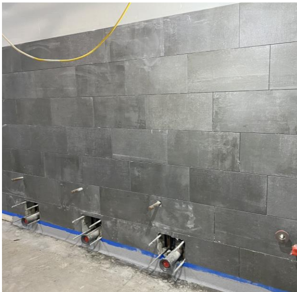
Wall tiling hung in the bathrooms in new addition.
