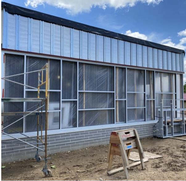
Aluminum frames installed for large windows in cafeteria addition.
