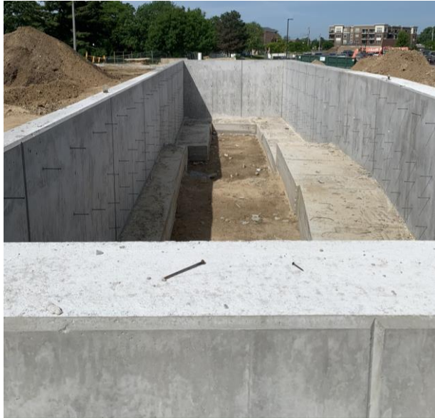
Tall planter poured on the north end of the new addition.
