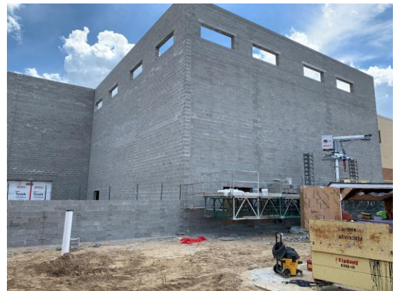
CMU firewall continuing west along the existing building.
