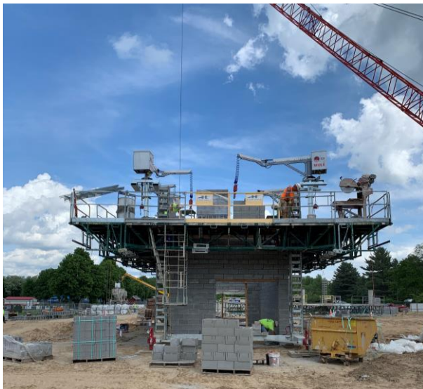
Masons working on Stair 2 with the help of the MULE system.
