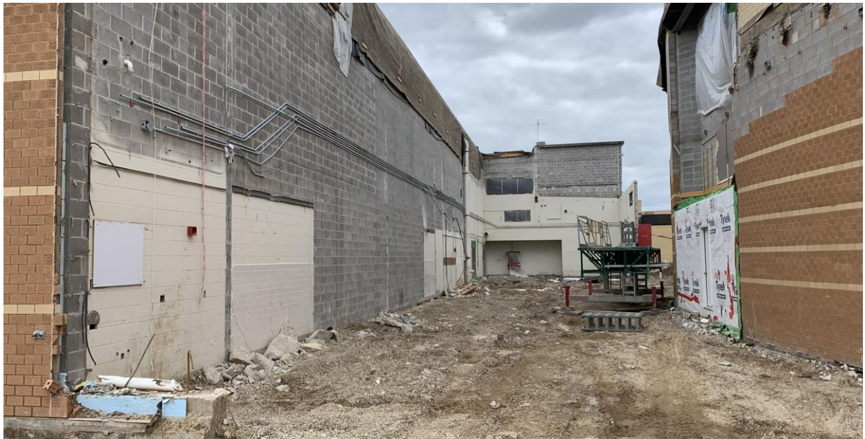
Demolition completed in the corridor in front of the PAC.
