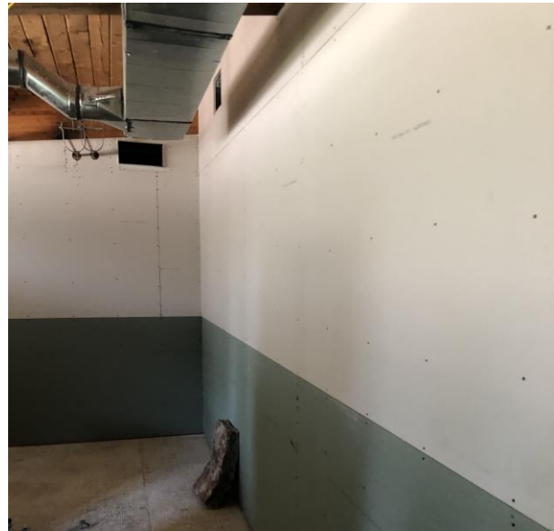
Drywall hung in the office and conference rooms.
