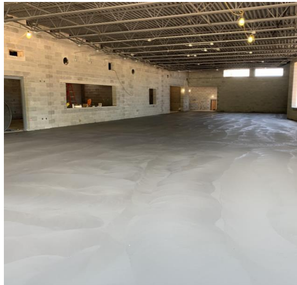
Slab-on-grade concrete poured in the cafeteria addition.
