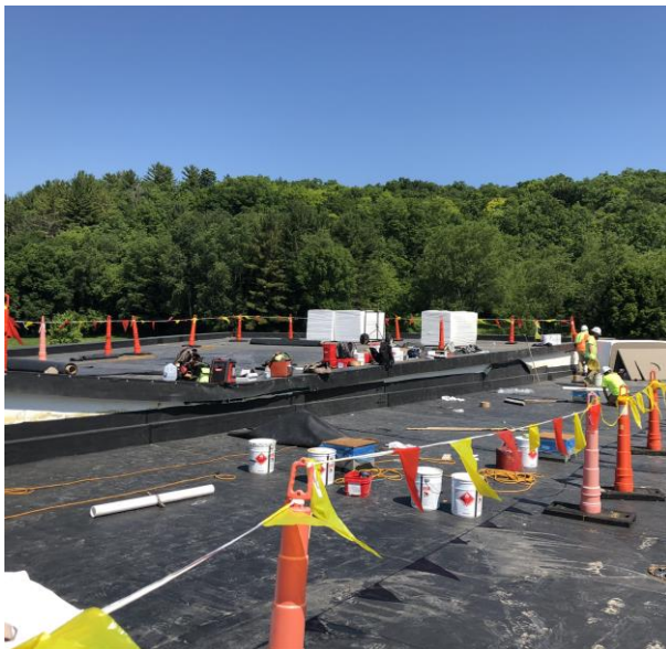
Roofing installation occurring on the new addition.
