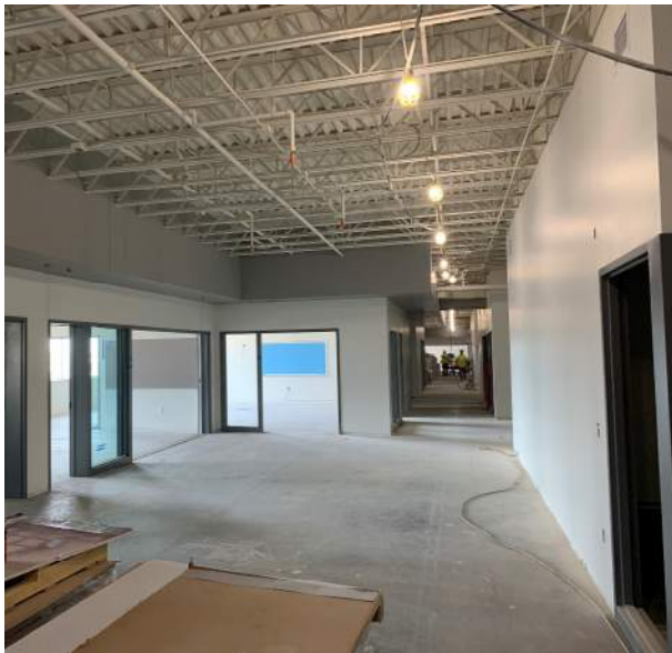
Area 1C hallway painting is nearing completion.
