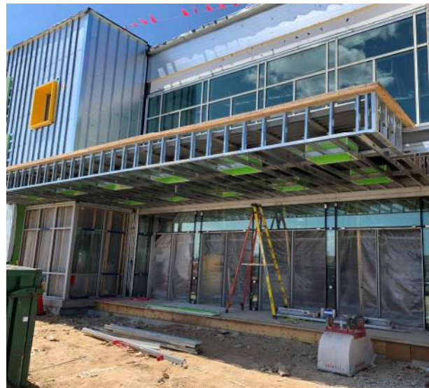
More glass being installed under the east canopy.
