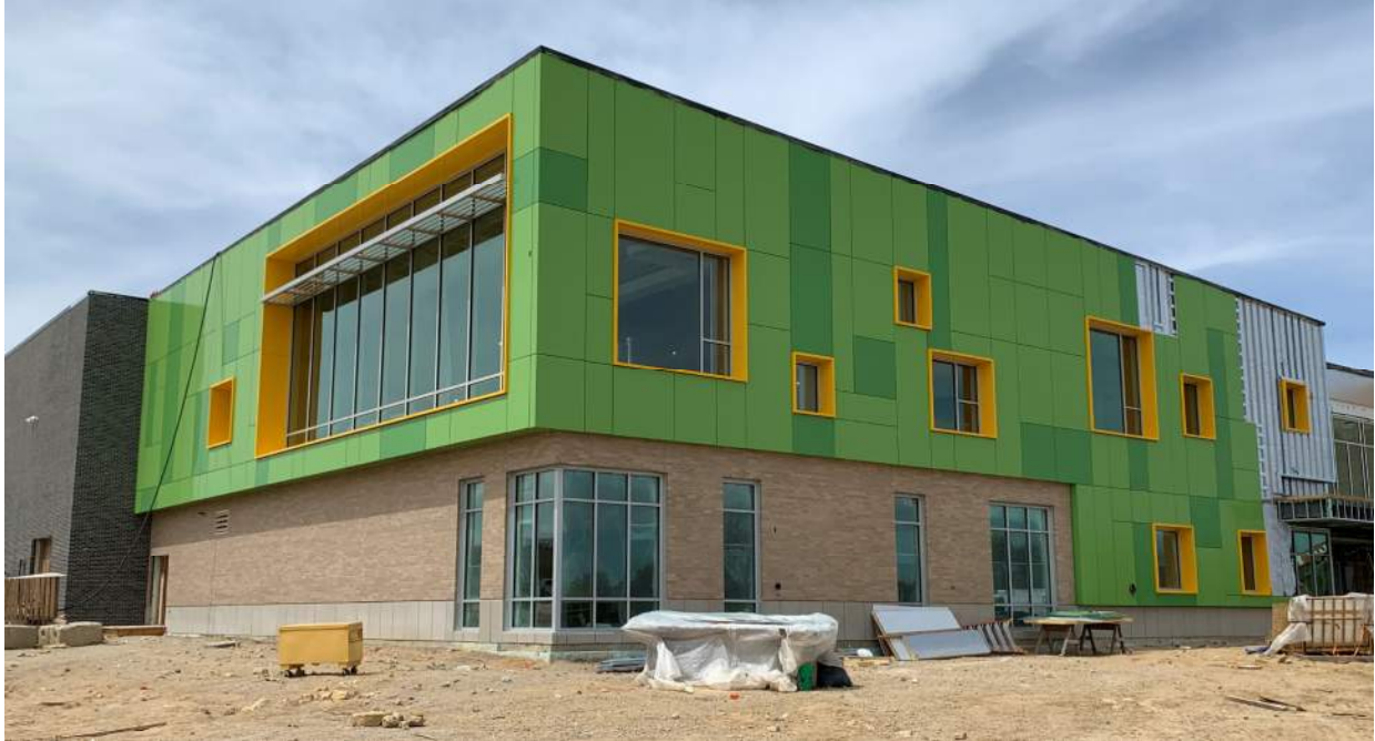
Exterior metal panel progress on the southeast side. The south side is completely finished with green panels, while the east side nears completion.
