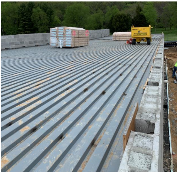
Metal decking installed above the steel trusses in preparation for roofing.
