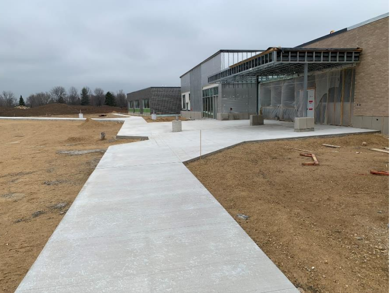
Below: Sidewalks poured outside the west side of the building.
