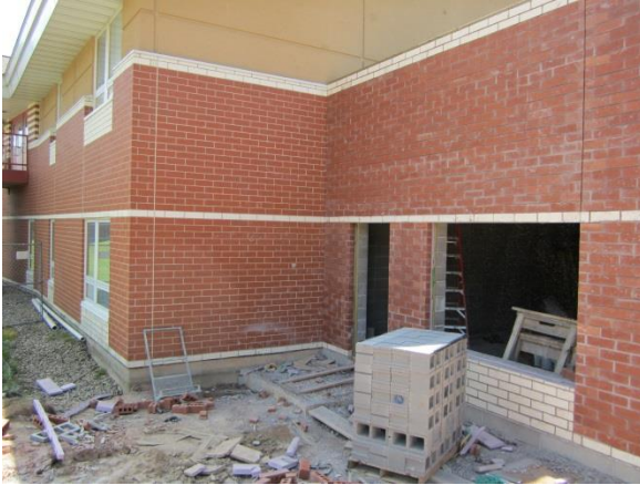
Brick is complete on the west addition.
