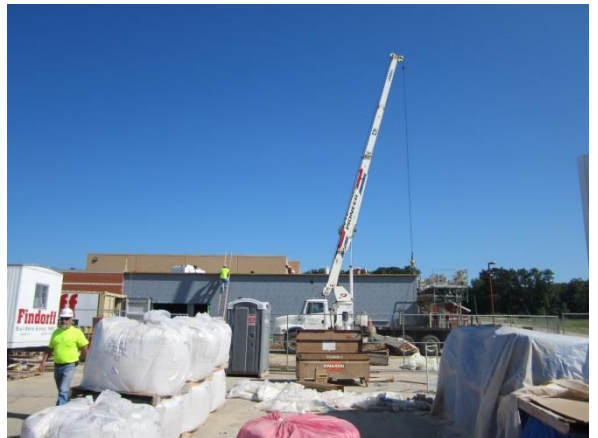
Installation of the roofing membrane has begun.
