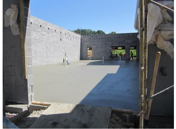
Both concrete slabs have been poured.
