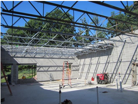
Steel roof framing is complete.
